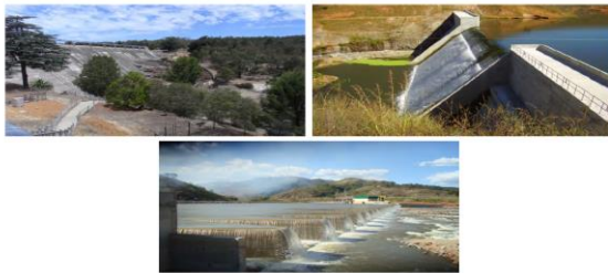
Fig. 1. Three samples of dam structures are shown here: 1) smooth waterfall; 2) flow over a stepped waterfall; and 3) a labyrinth [25]
