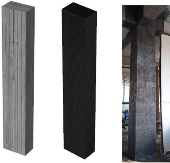
Fig. 10. Before/after reinforcement and application example
