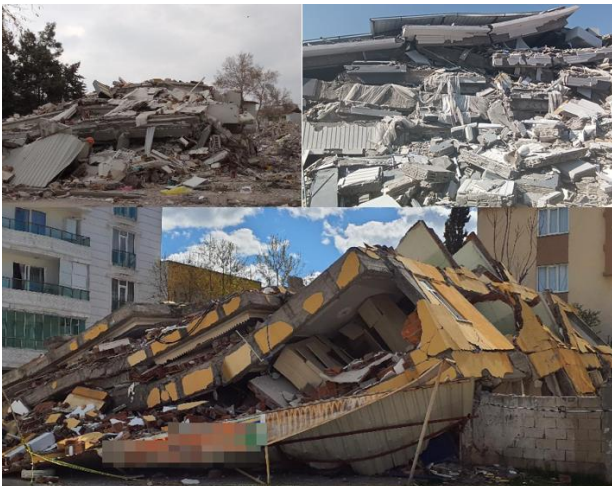
Fig. 1. Totally collapsed R/C buildings.
